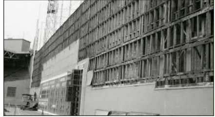
After the 1975 season, the original tin facing of the Green Monster was stripped off.
