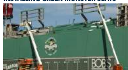
INSTALLING GREEN MONSTER SEATS
